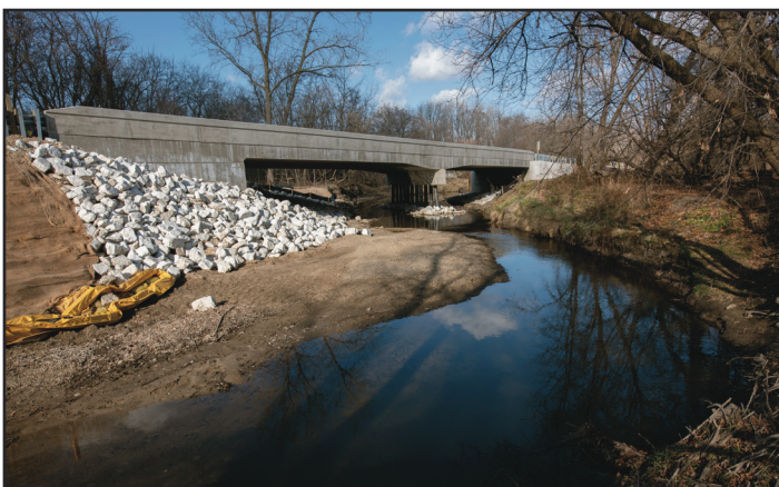
The 13th Avenue bridge over the Pike River has been repaired.
