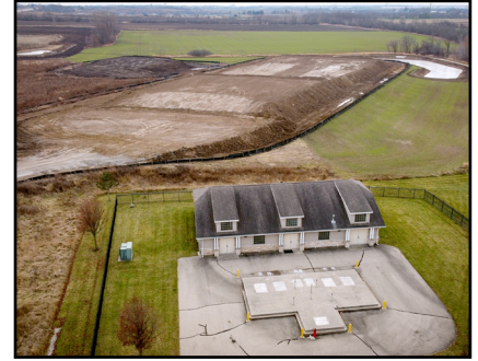
Soil is being brought to the Willow Creek site.
