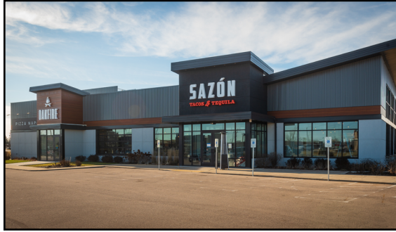
The Oakfire Pizza restaurant is being split in two.
